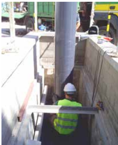
Figure 4: Installation of a suction flow control device (SFCD) in a water well.
